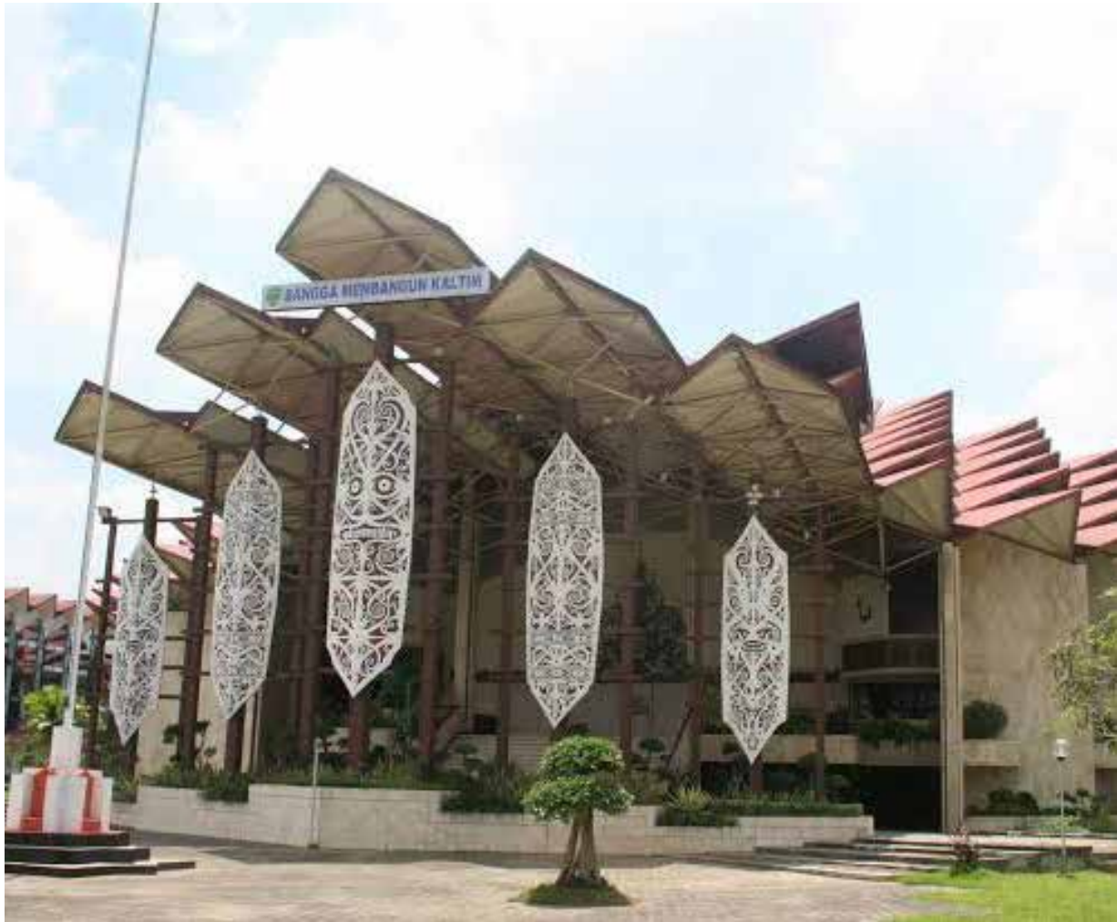
Gedung DPRD Kaltim (ist)
